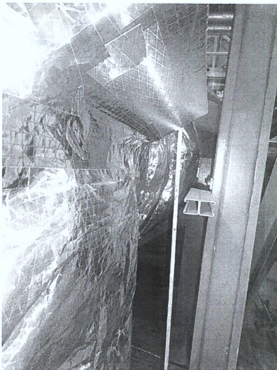
Figure 4 Missing Support on Air Line Hard Pipe to Valve 1Z41-F009B
