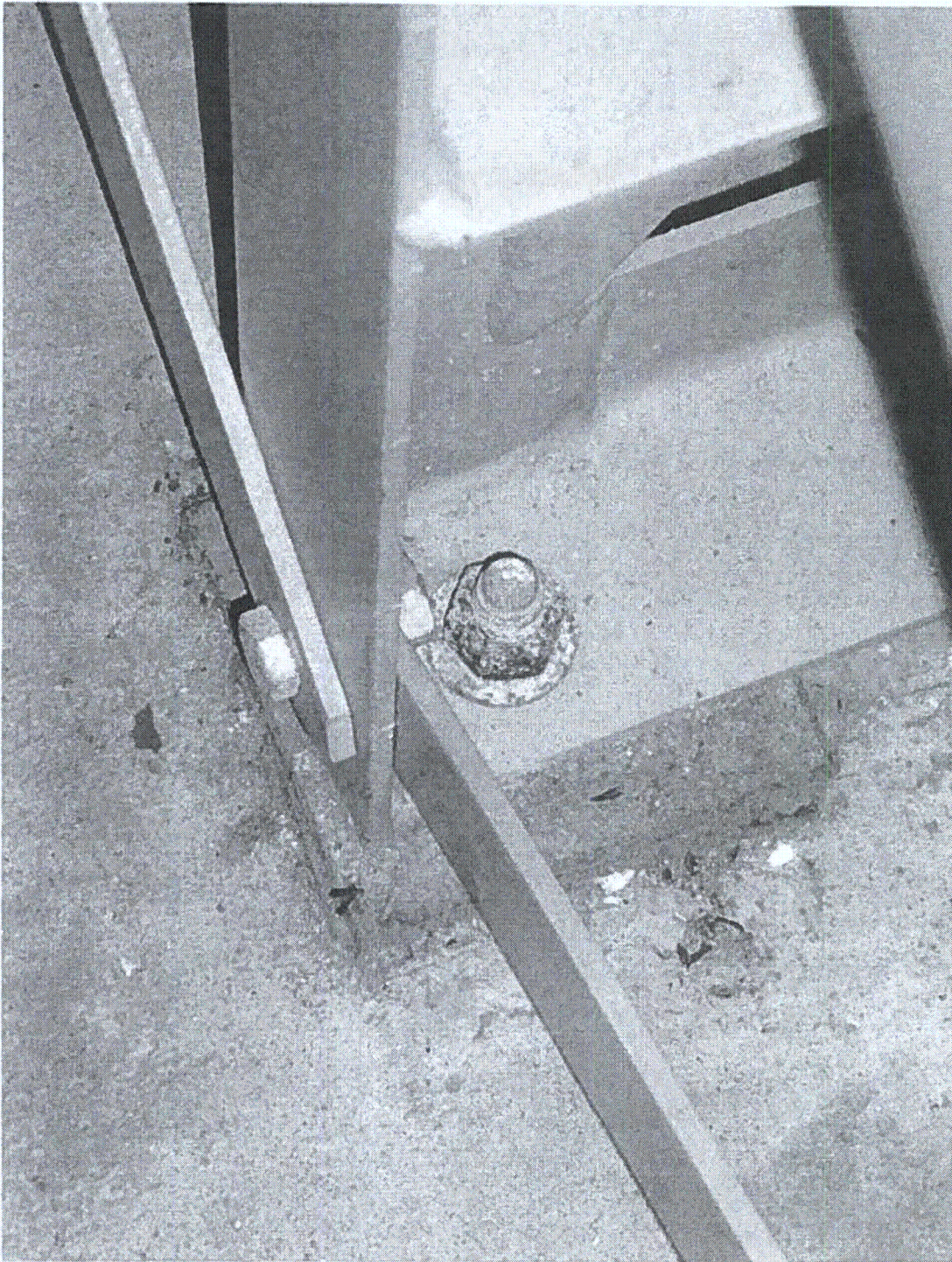
Figure 3 – Surface Oxidation on Anchor Bolt (1R42-S002B)
