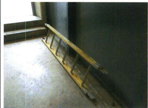
Note: unrestrained ladder by the door at the south corner of the room.
