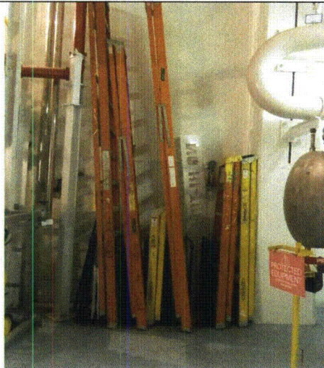
Note: Unrestrained ladders in a rack
