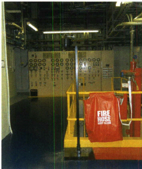
Note: Camera on post with unsecured base plate
