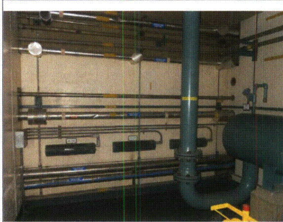
Note: View of wall and conduits
