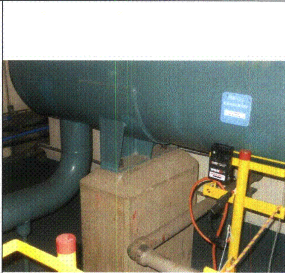
Note: View of exchanger pedestal and anchor bolts
