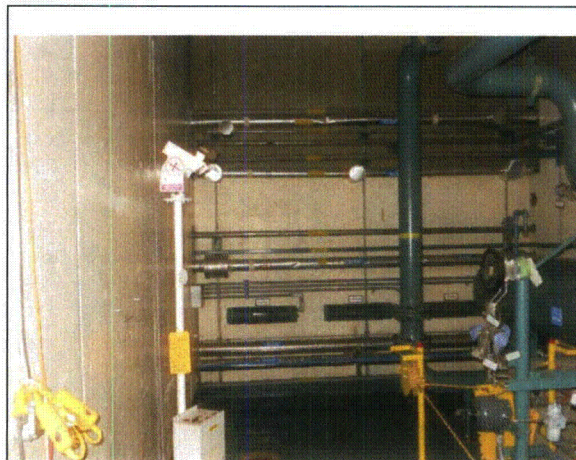
Note: View of rear wall
