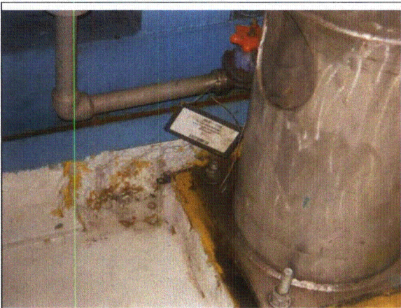
Note: Excavated area of pedestal
