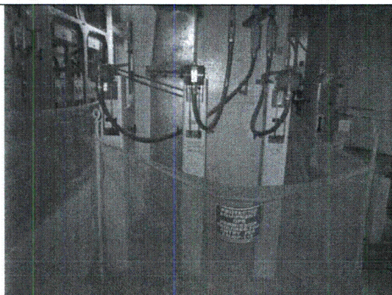
Note: General view of the area
