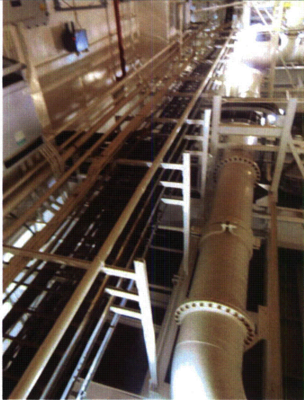
Area # Intake, 8-7, CAL-ISPR-INT1 8-16-12 204
