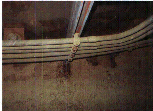
Area # Yard, 45, CAL-TKFROOM 8-15-12 012
