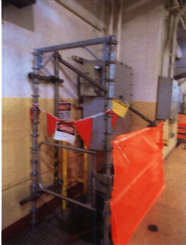
Area # Intake, 8-7, CAL-ISPR-INT1 8-16-12 208
