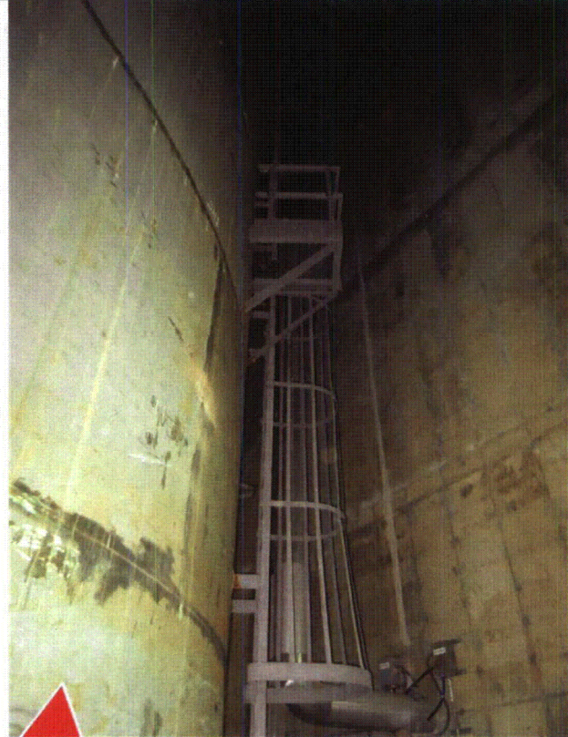
Area # Yard, 45, CAL-TKFROOM 8-15-12 010
