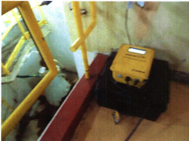
Area # Intake, 8-7, CAL-ISPR-INT1 8-16-12 202
