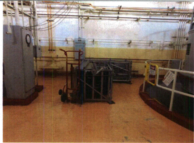
Area # Intake, 8-7, CAL-ISPR-INT1 8-16-12 197
