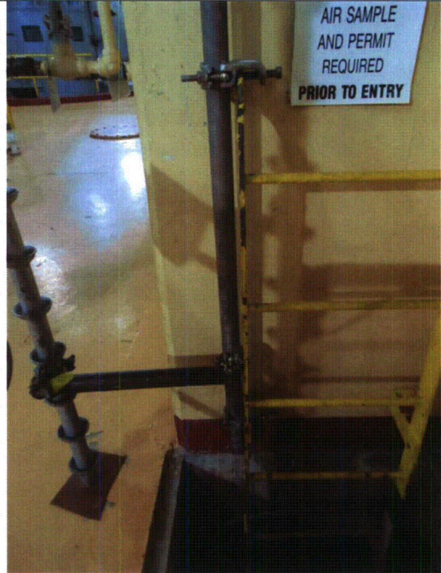
Area # Intake, 8-7, CAL-ISPR-INT1 8-16-12 207
