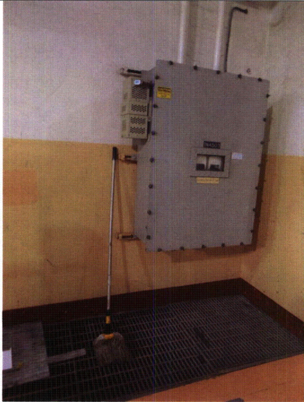
Area # Intake, 8-7, CAL-ISPR-INT1 8-16-12 196
