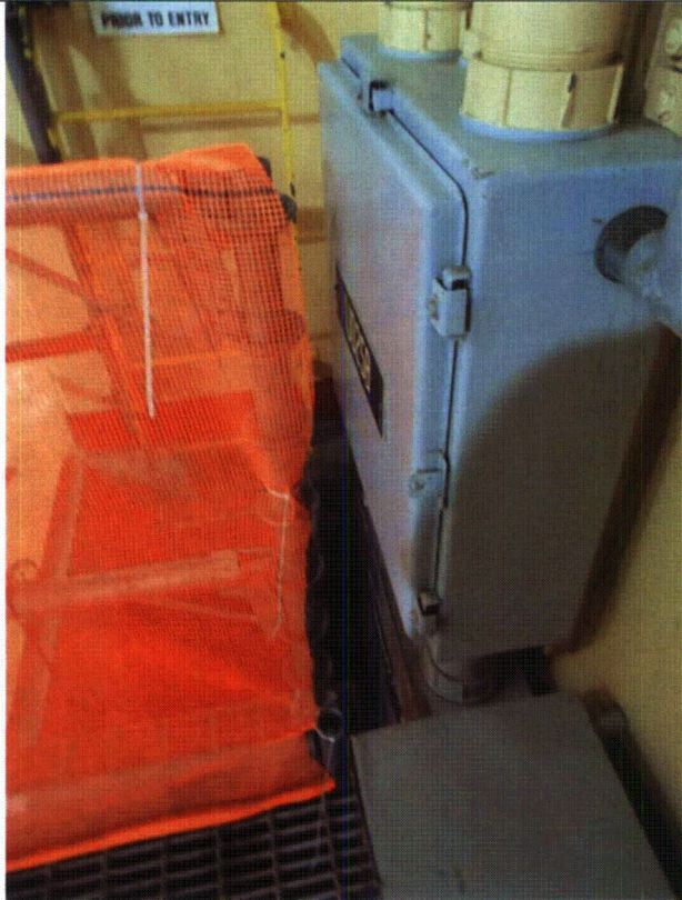
Area # Intake, 8-7, CAL-ISPR-INT1 8-16-12 206
