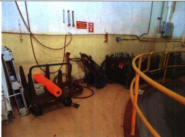
Area # Intake, 8-7, CAL-ISPR-INT1 8-16-12 194
