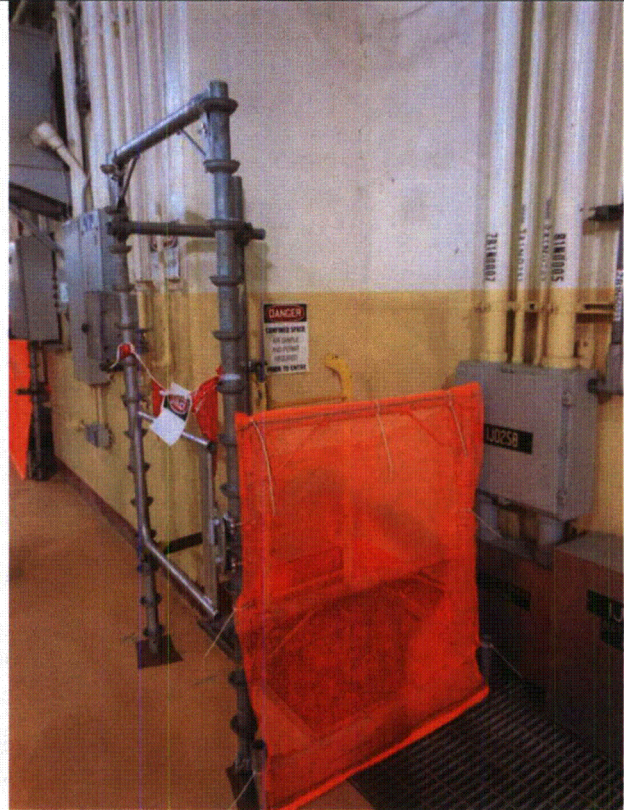
Area # Intake, 8-7, CAL-ISPR-INT1 8-16-12 205
