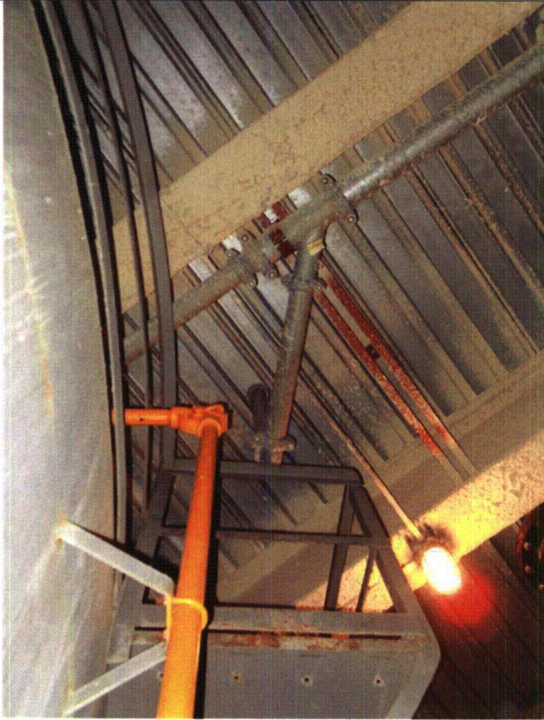
Area # Yard, 45, CAL-21FOSTBLDG 8-13-12 085
