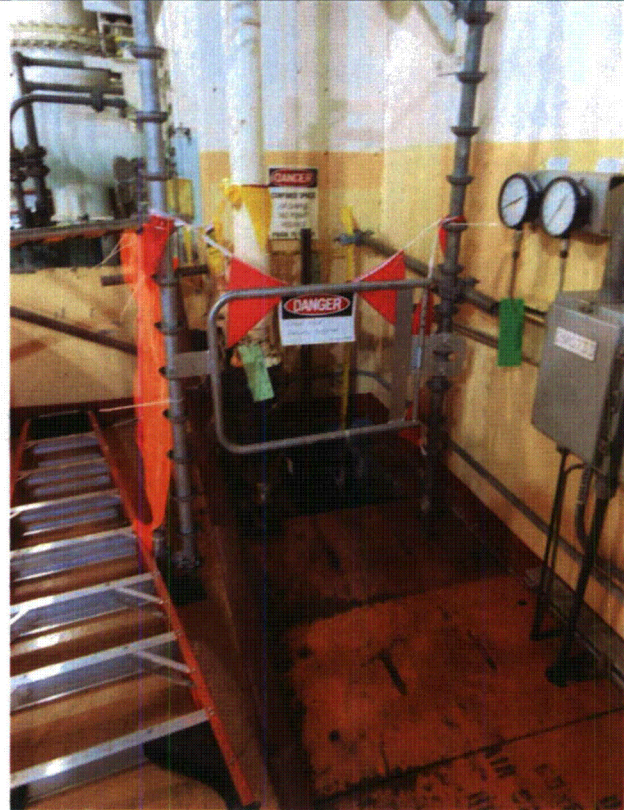
Area # Intake, 8-7, CAL-ISPR-INT1 8-16-12 212
