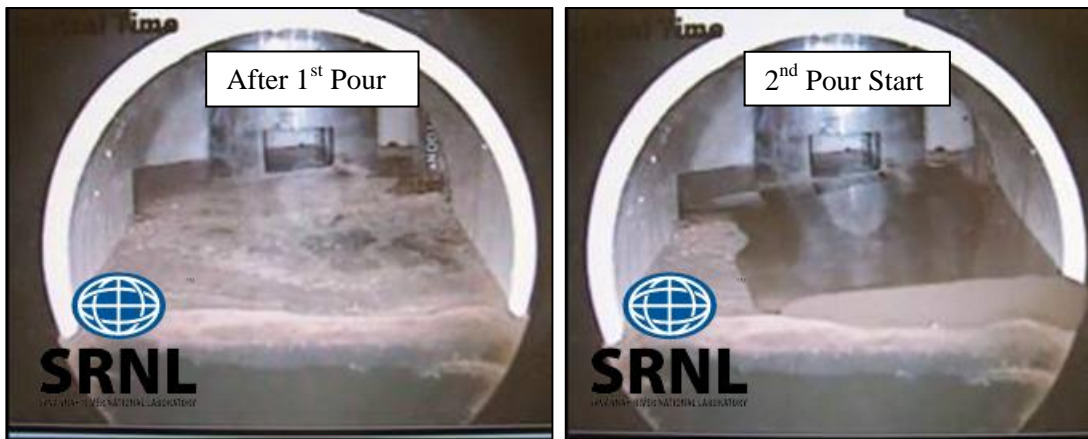
Figure 3-2. Site Port #5 View Between Pours.
