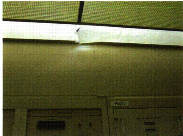
1PM05J (AWB CRACKED CEILING TILE) Byron 1 & 2 010
