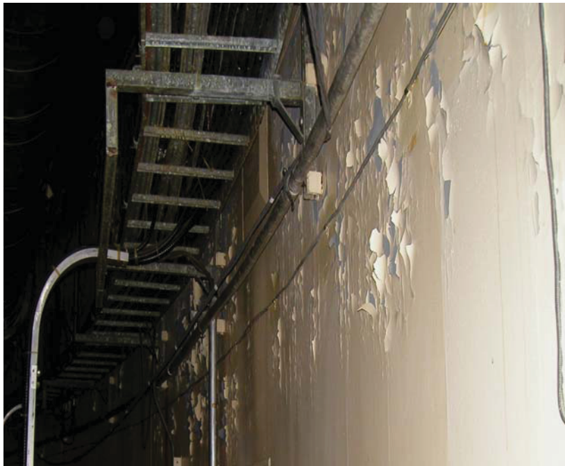
Figure 4 Example of Coatings Degradation at Oconee
