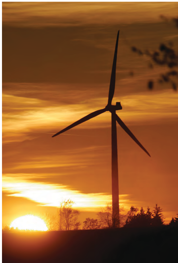
Photo courtesy of Maple Ridge Wind Farm
