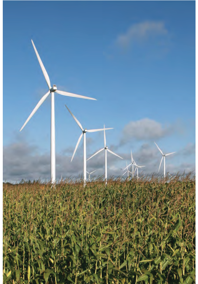
Photo courtesy of Maple Ridge Wind Farm
