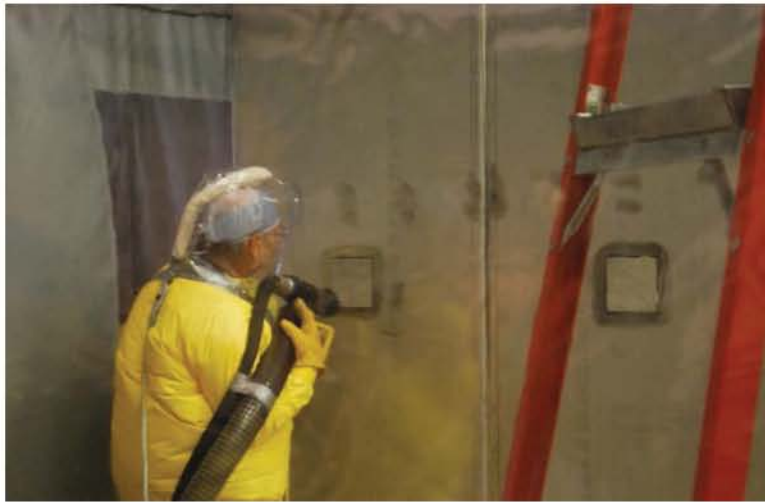
Figure 3-3. Operator applying Blast N'Vac to concrete coupon.
