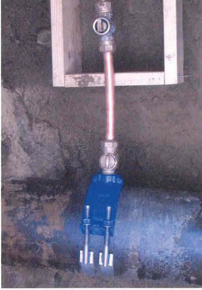
Plan view of Saddle clamp and 1" branch to MTF
