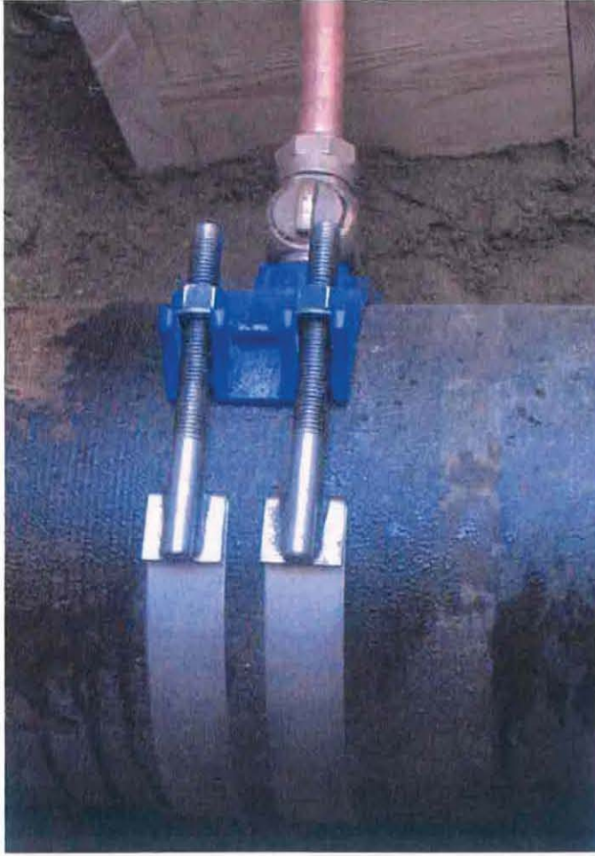
10" double strap Saddle + 1" Branch to MTF
