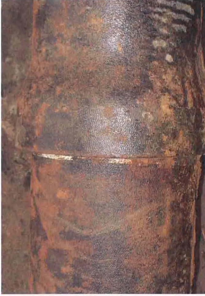
10" CW piping Bell & Spigot Joint
