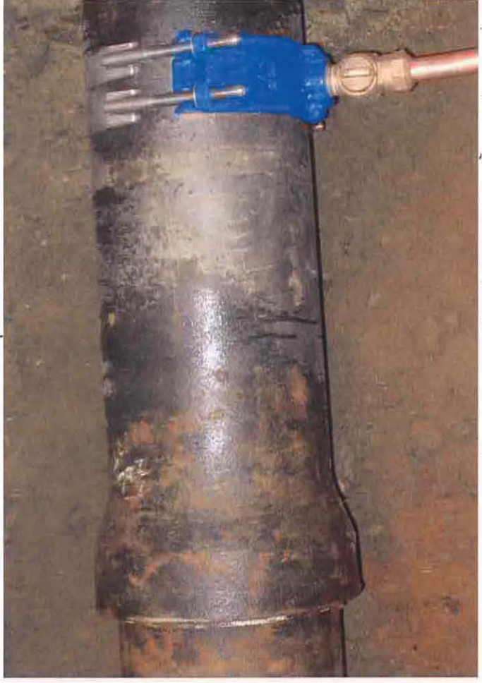
Plan view of Saddle clamp and 1" branch to MTF
