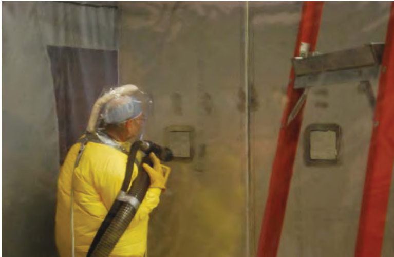
Figure 3-3. Operator applying Blast N'Vac to concrete coupon.
