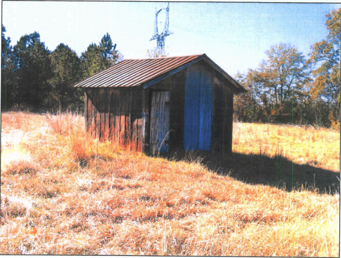
Figure 57. 51160, smokehouse, view southwest.
