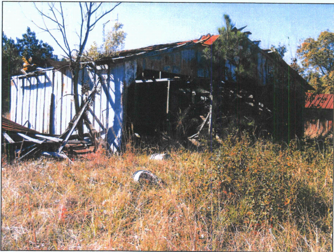
Figure 56. 51160, barn 2, view southwest.
