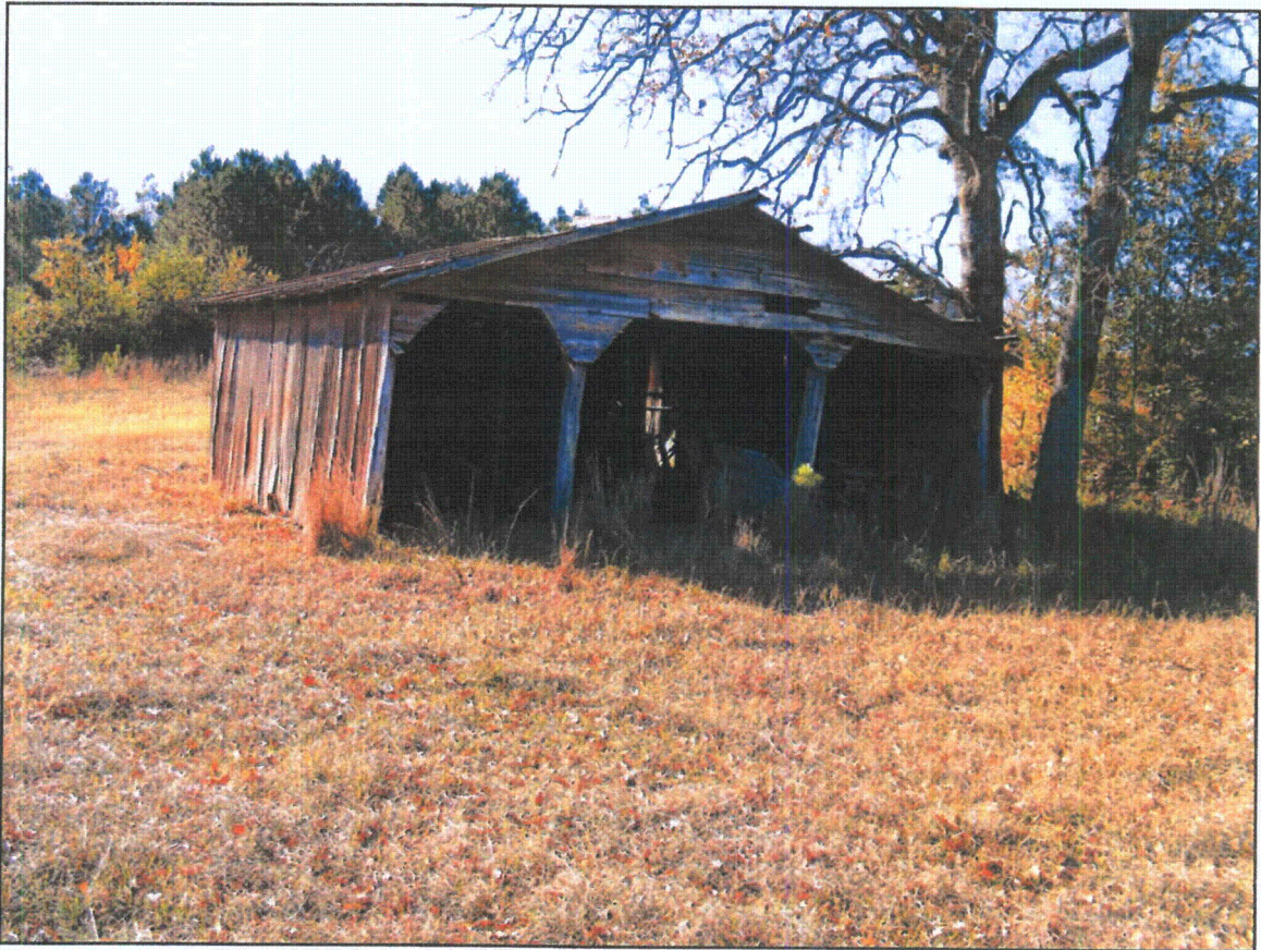
Figure 55. 51160, barn 1, view southwest.
