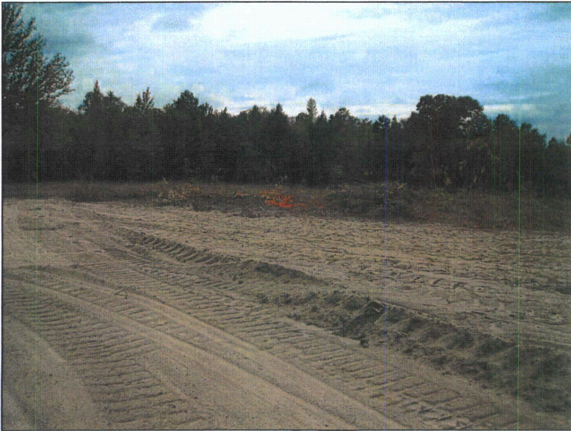
Figure 32. General view of 9JF338 site area.
