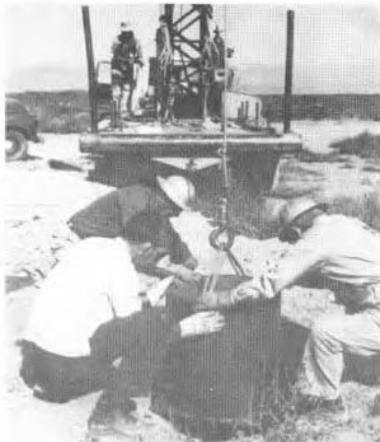
Figure 5-5. TYPICAL PLACEMENT OF PROTECTIVE CANISTER.
