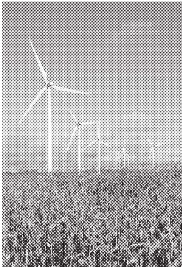
Photo courtesy of Maple Ridge Wind Farm
