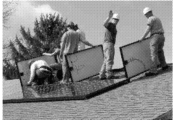
PV system installation
