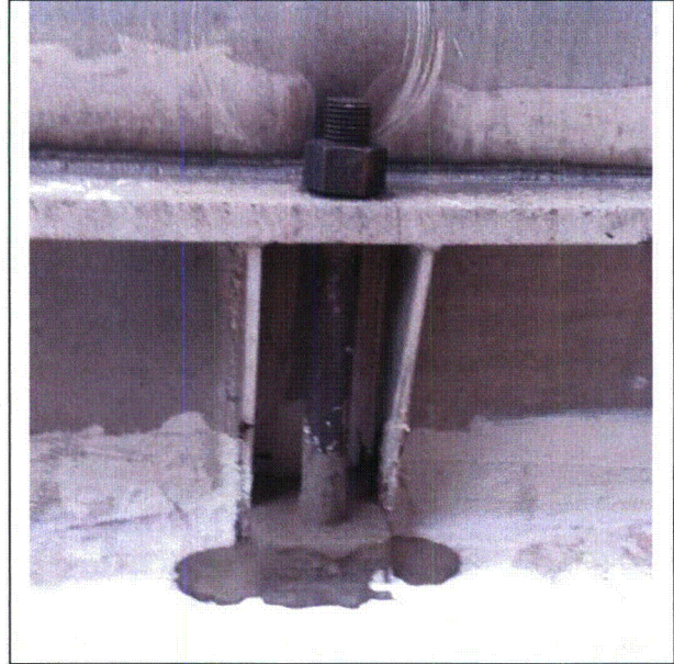
Note: Tank T-58 Anchor Bolt. 1 of 52
