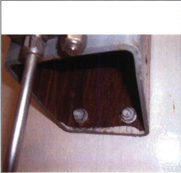
Note: PT-0741DD Lower Conc. Anchors
