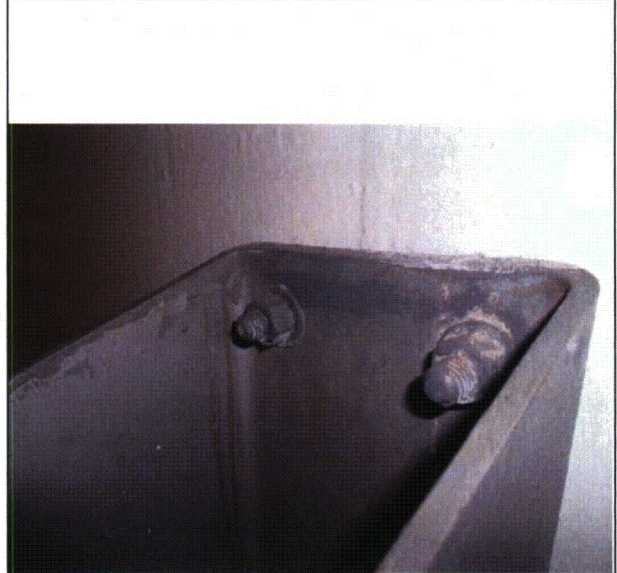
Note: PT-0741DD Upper Conc. Anchors
