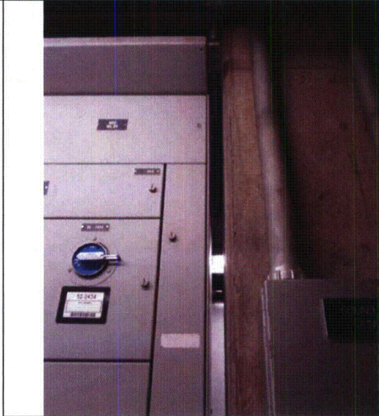
Note: Nearby Concrete Column
