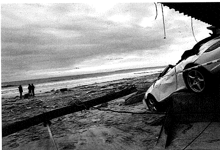
The boardwalk has been washed away in Rockaway.
