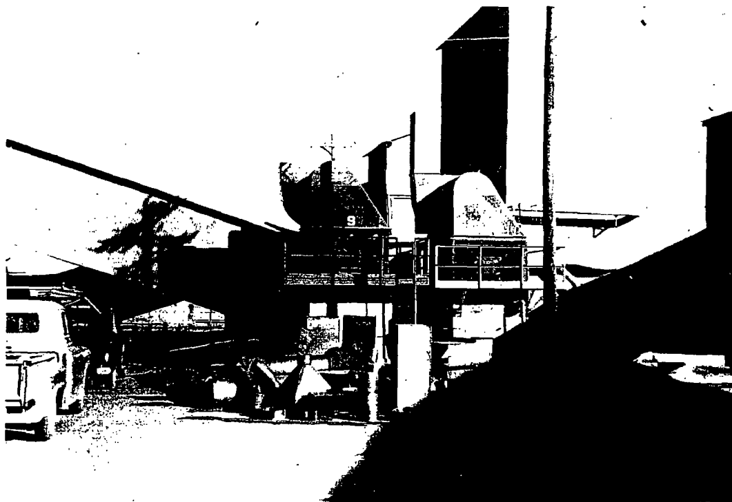
4. Installation of dust collection equipment in crushing and sampling area.
