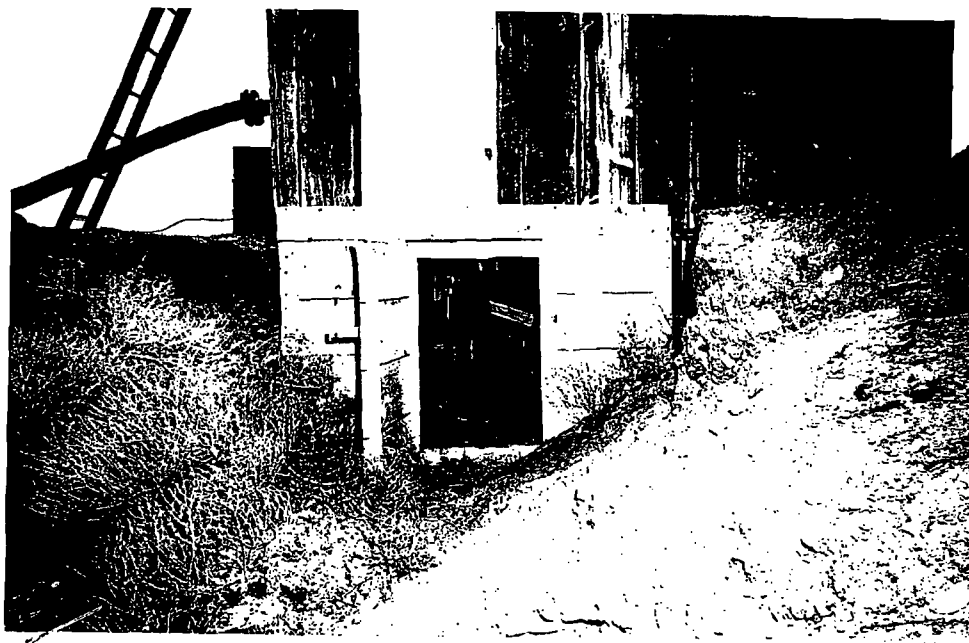
14. Lower portion of disposal well building showing point where pipe enters ground.
