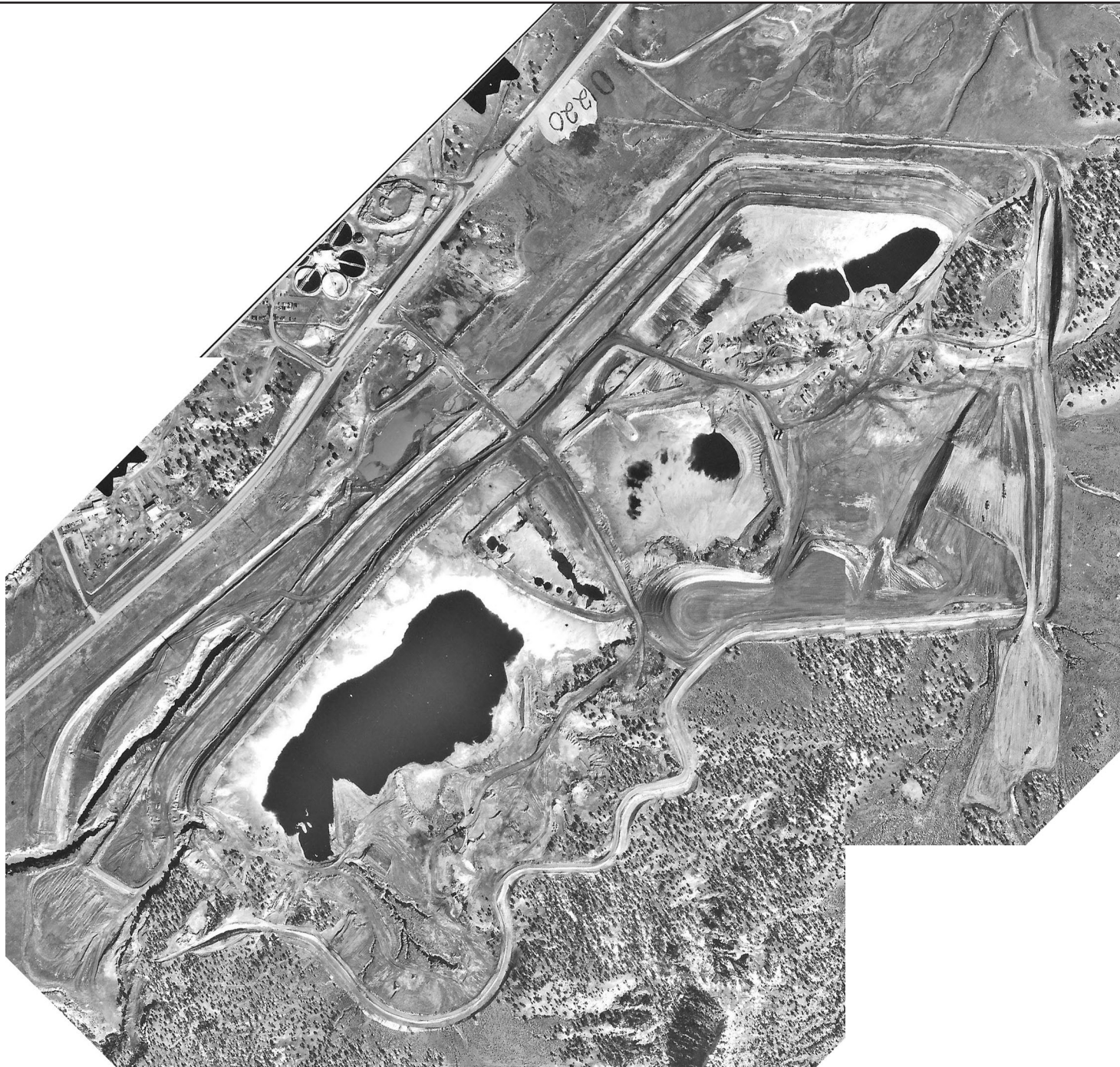
FIGURE B-5 Collage of October 23, 1979 aerial photographs, source UNC
