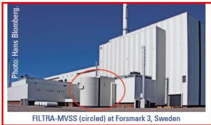
One example: Westinghouse FILTRA-MVSS (multi-venturi scrubber system) is described as a passive, self-regulating system for filtered pressure relief of BWR/PWR reactor containments<sup>12</sup>. The system is passively actuated by means of a rupture disc. A typical design basis for the system is a total loss of AC power for 24 hours leading to loss of core cooling
