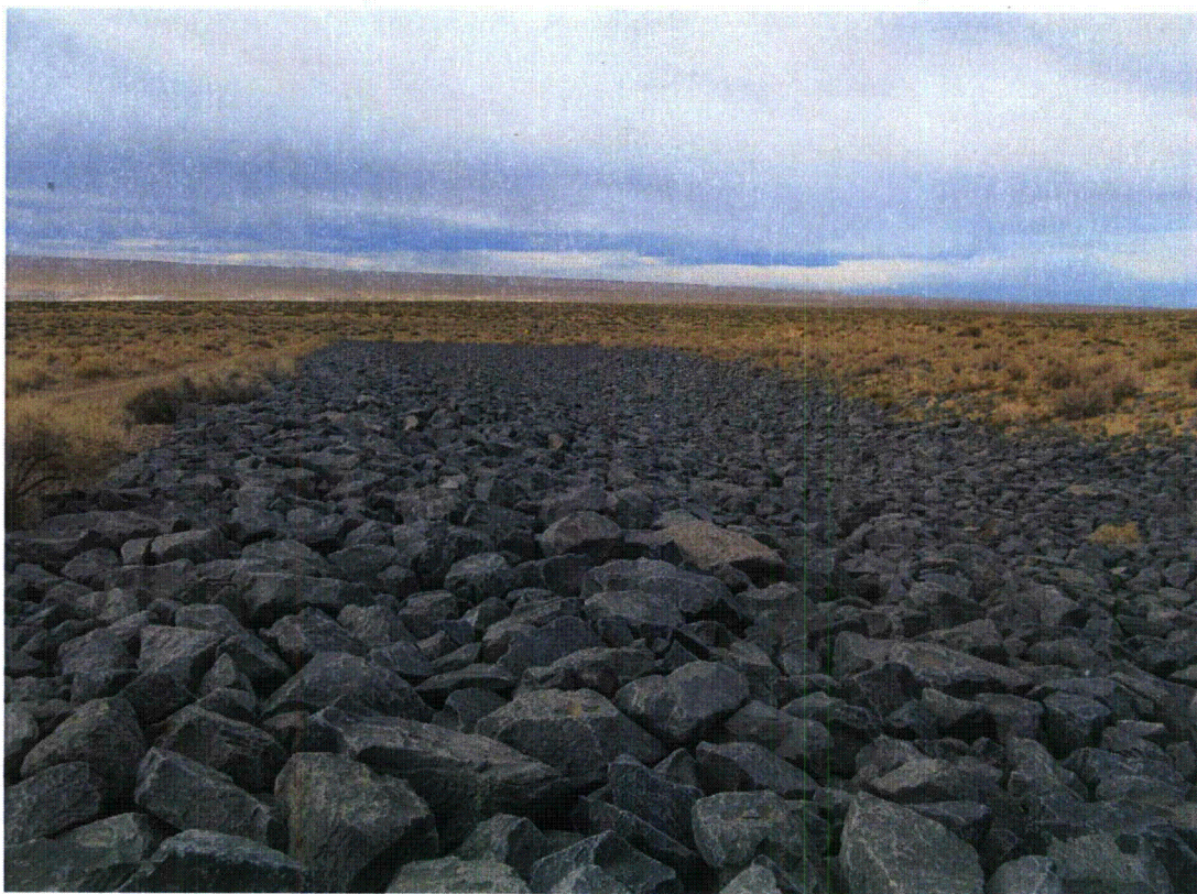
TUB 4/2011. PL-6. Diversion channel on the west side of the site.
