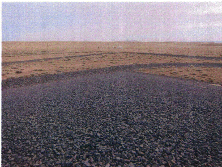
Figure 2: Diversion Ditches as Seen from Top of Impoundment
