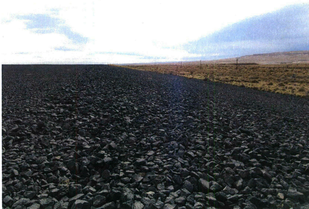
TUB 4/2011. PL-2. South side slope of the disposal cell cover.
