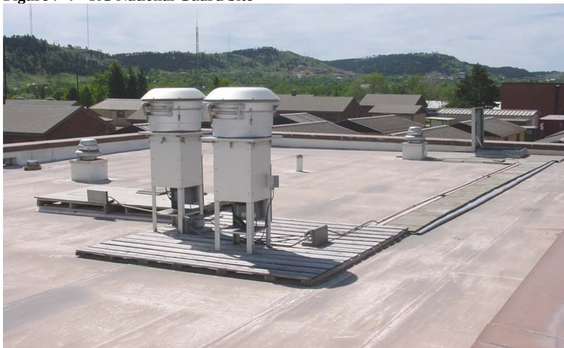
Figure 7-4 – RC National Guard Site
