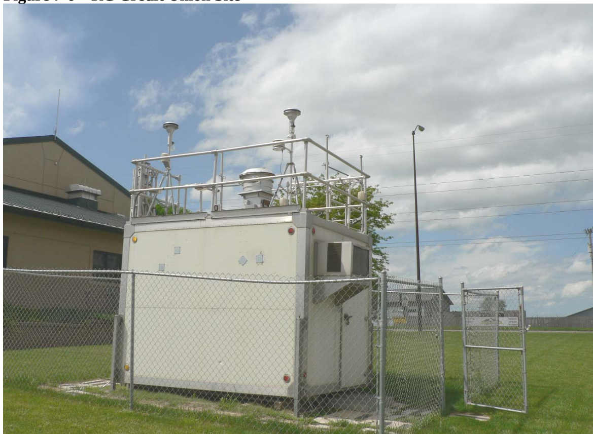
Figure 7-6 – RC Credit Union Site
