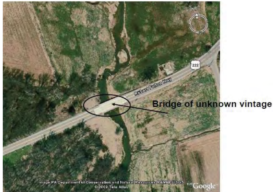
Figure 6-16 Bridge along Robert Fulton Highway
