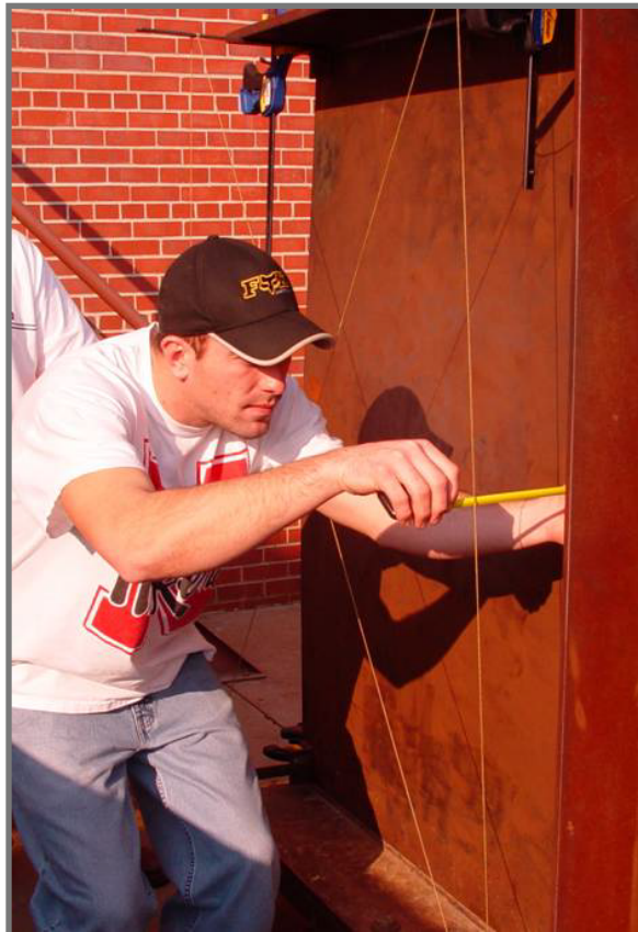
A fabricated girder is being inspected for distortion, sweep and web flatness
