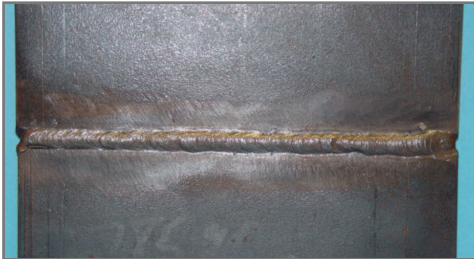
Slag rolled into toe of weld
