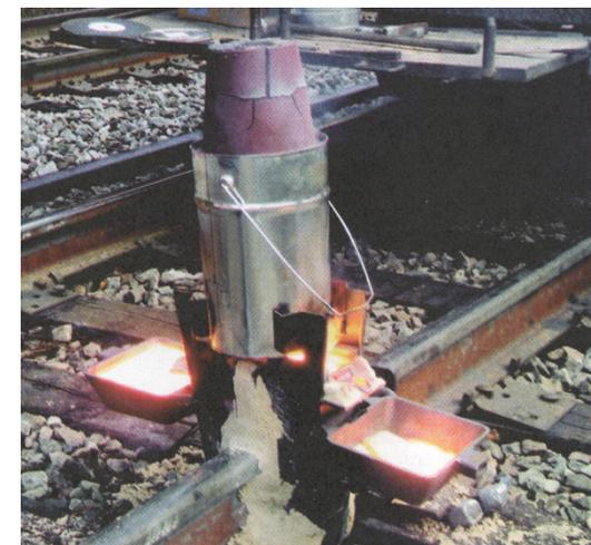
Thermite Welding of rails
