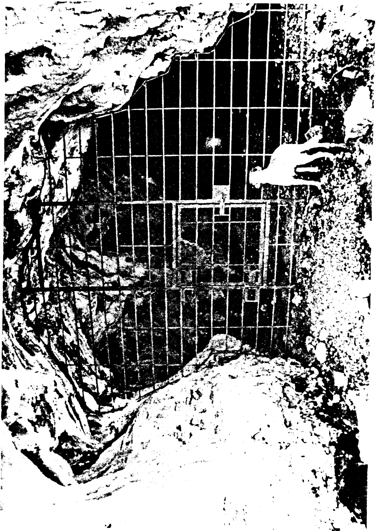
FIGURE 6: Great Scott Cave gate erected by the Missouri Department of Conservation (Photo Credit - R. Clawson).
