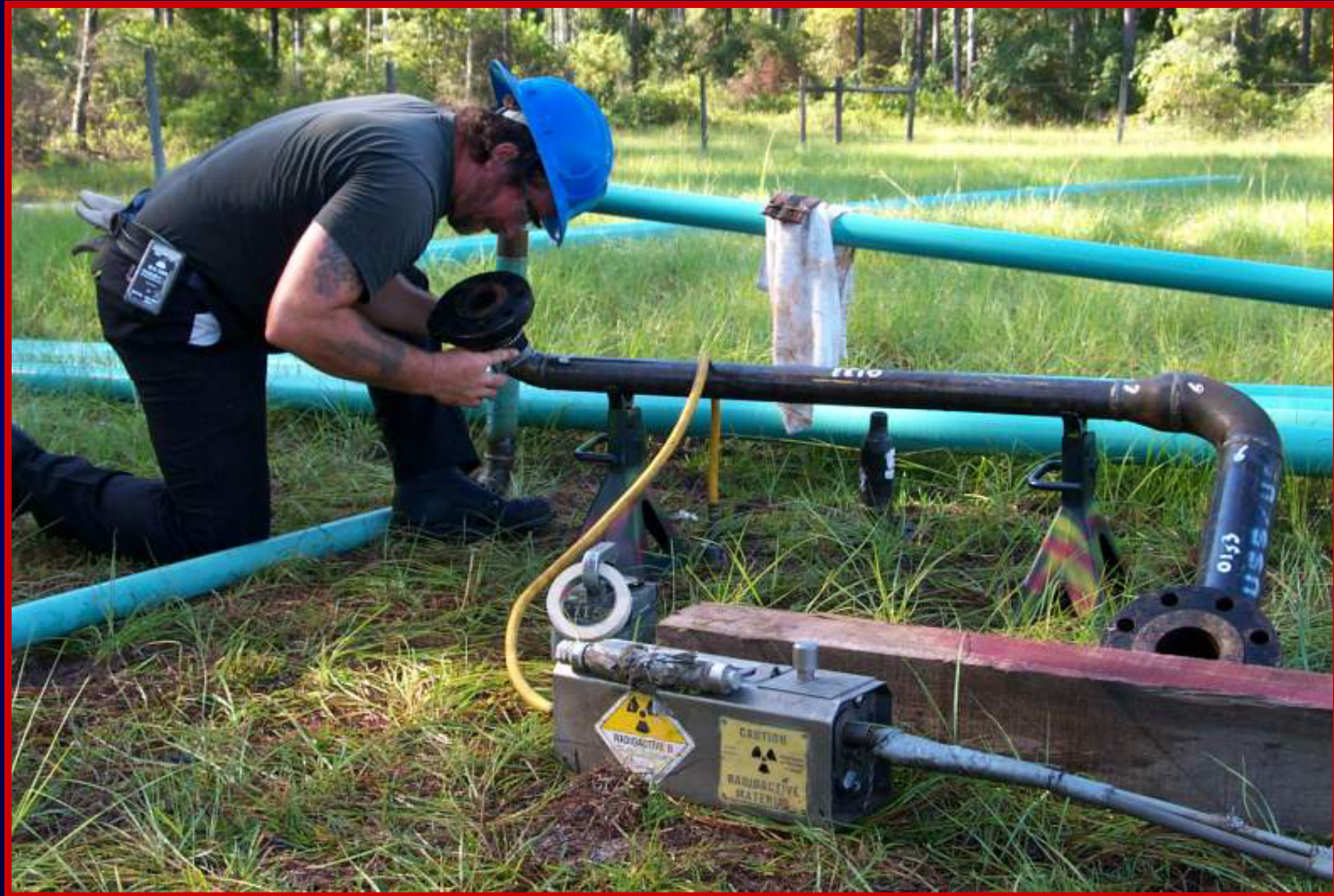
RT of gas pipeline - Pensacola, FL
