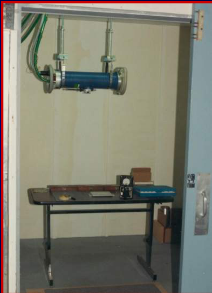
Vault equipped with X-ray machine
