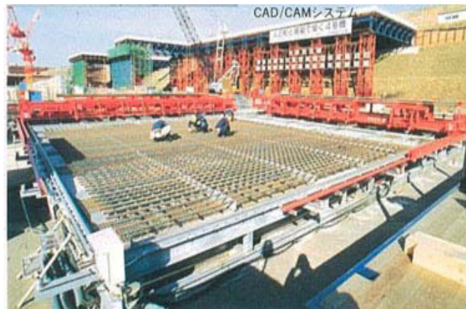
FIG. IV-13. An automatic rebar assembly machine at Kashiwazaki Kariwa-7 in Japan.
