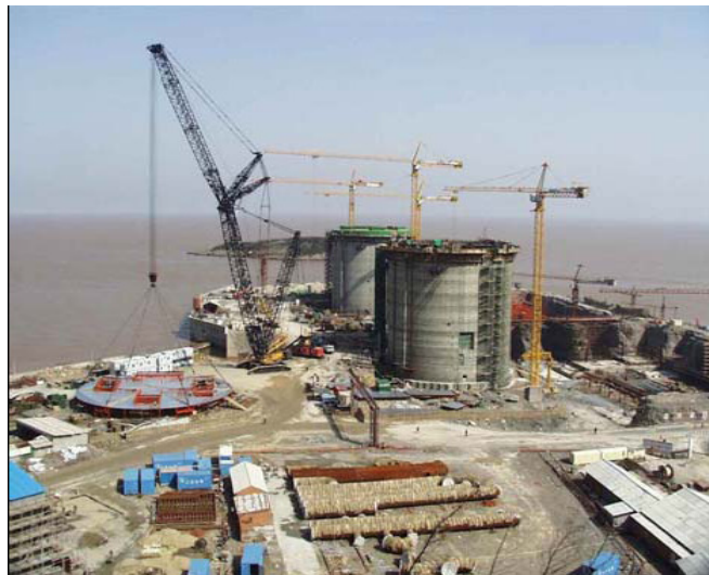
FIG. IV-1. Very heavy lift crane at Qinshan, China.
