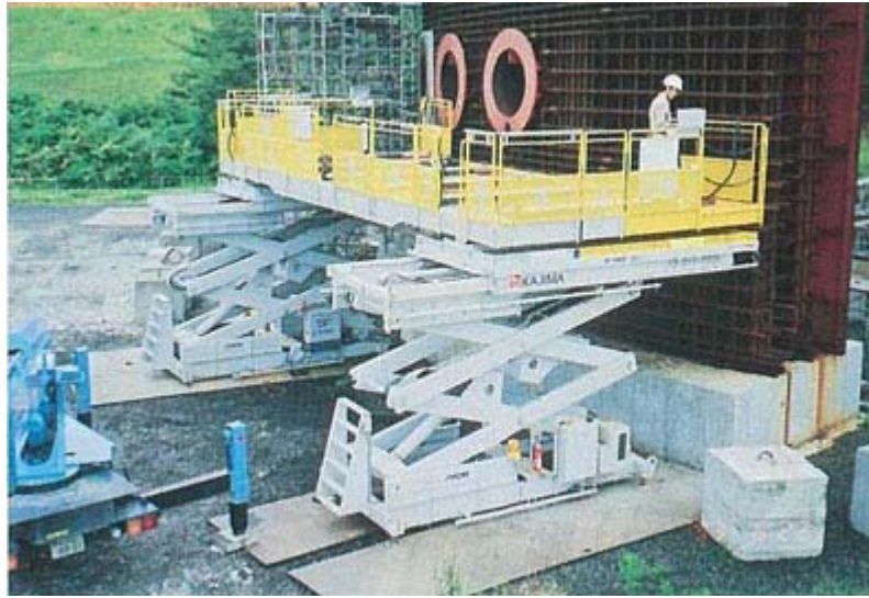
FIG. IV-12. An automatic scaffold and horizontal rebar feeding machine at Kashiwazaki Kariwa-6 in Japan.
