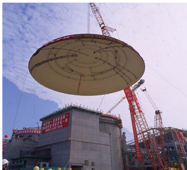
FIG. IV-8. Lifting the dome module into place at Lingao-4 in China.
