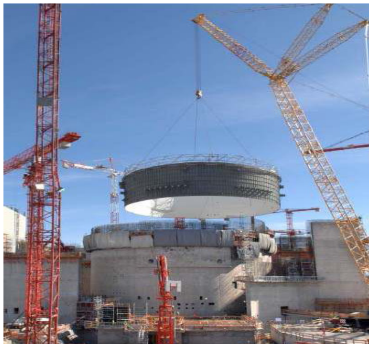
FIG. IV-3. Lifting the containment liner double rings at Olkiluoto-3 in Finland.
