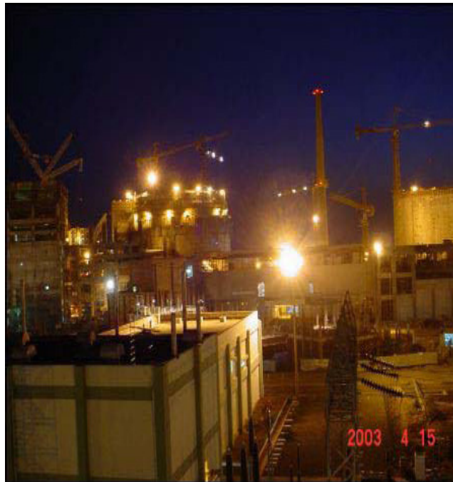
FIG. IV-14. Night view of site activities at Tarapur-4 in India.
