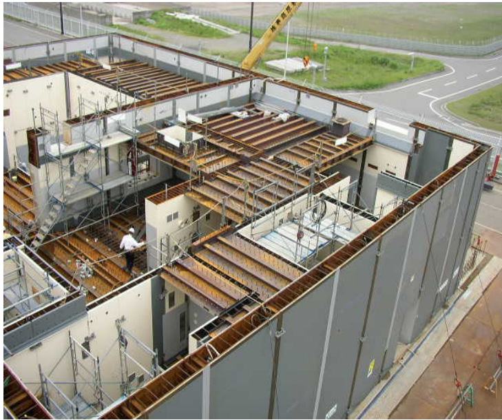
FIG. IV-11(b). Steel Plate Reinforced Concrete
