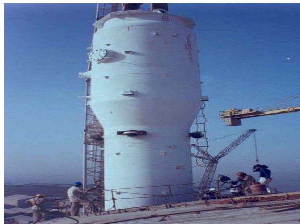
FIG. IV-5(a) and IV-5(b): Installing a steam generator at Tarapur-3, India.
