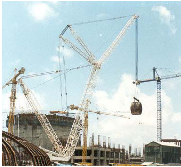
FIG. IV-6. Lifting the calandria at Tarapur-3 in India.
