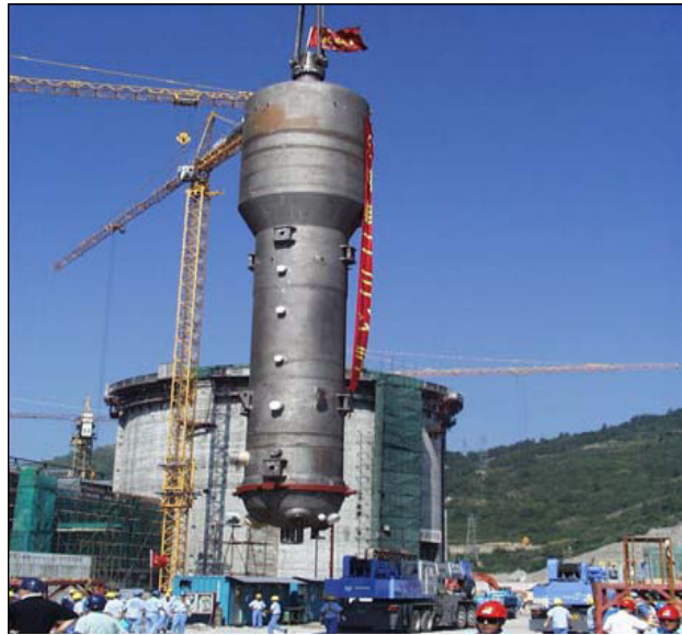
FIG. IV-2. Installing a steam generator at Qinshan 3-1 in China
