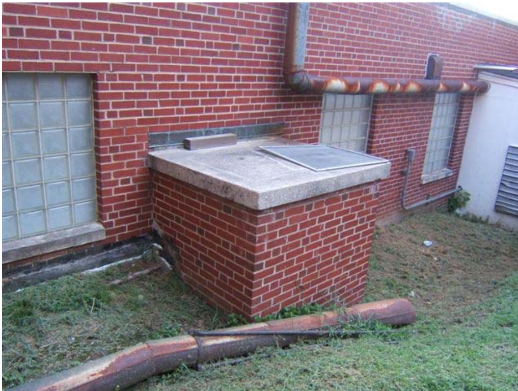
Portion of old Nuclear Medicine Pharmacy vault. View from South
