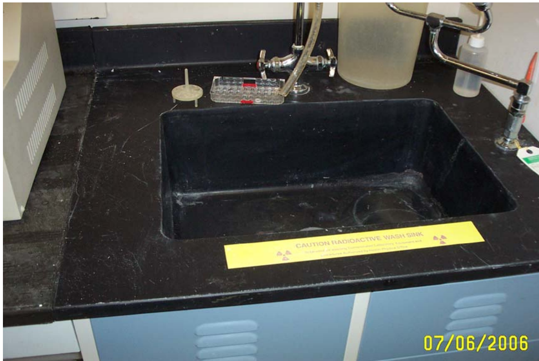
Example of Sink used for RAM use and disposal purposes
