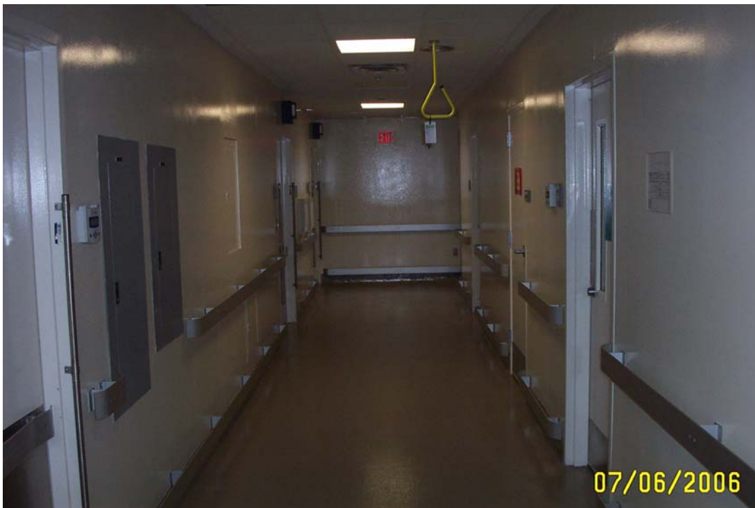
5 th Floor Animal Research Area. Completely renovated from original condition
