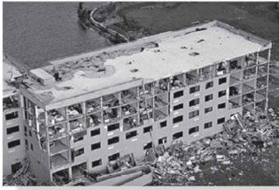
Figure: FG01_09UN Hurricane winds caused this damage to a condominium in Miami, Florida.
