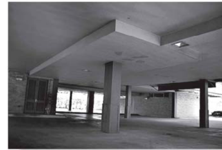
Figure: FG01_07UN Shown is a typical example of an interior building column. The live load office floor loading it supports can be reduced for purposes of design and analysis.
