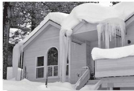
Figure: FG01_10UN Excessive snow and ice loadings act on this roof.
