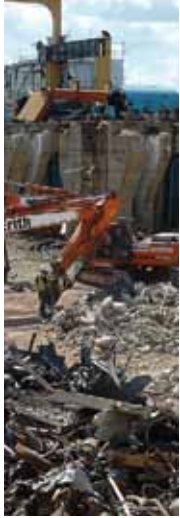
Bradwell turbine hall demolition
