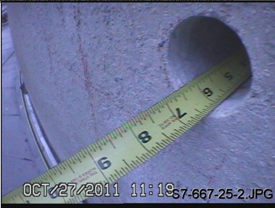
Picture No. 6- Davis-Besse Shield Building Core Bore Location S7-667-25-2
