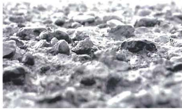
Fig. 3: Surface prepared by hydrodemolition has a rough irregular profile with protruding aggregate and is excellent for creating a mechanical bond
