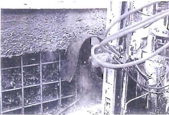
Fig. 15: Partial depth removal on a retaining wall
