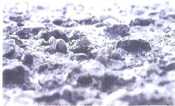
Fig. 12: Scarified surface with 1 in. aggregate
