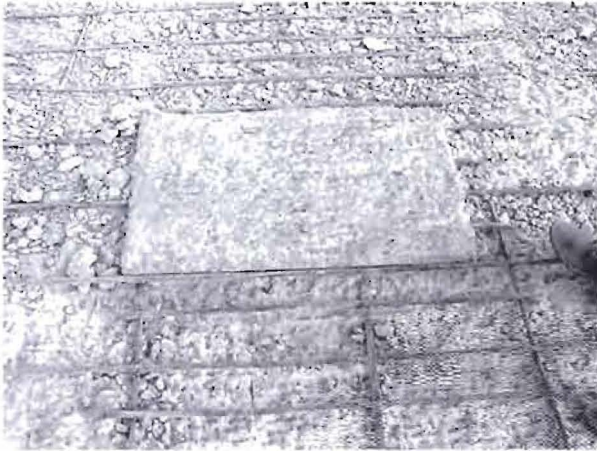
Fig. 20: High-strength repair area within the hydrodemolition area
