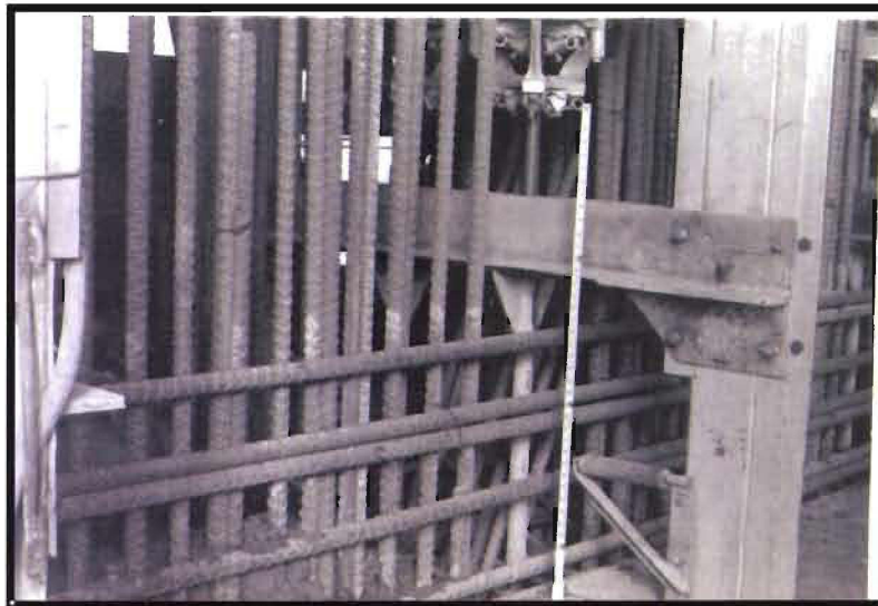
Figure 3: High Density of Reinforcement at Outer Rebar Mat (Photo during Construction)
