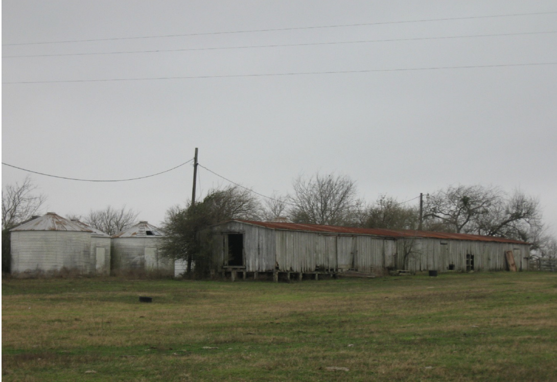
Figure 281. Street Number Unavailable, Cushman Road, Barn 7, looking south-southeast.
