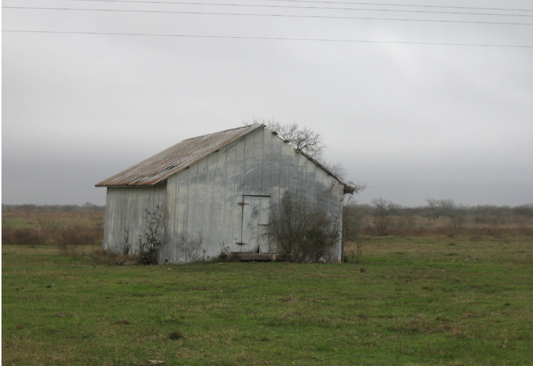
Figure 278. Street Number Unavailable, Cushman Road, Barn 5, looking north-northeast.
