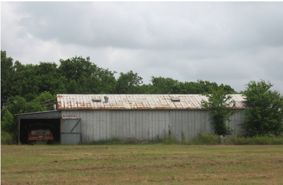
Figure 274. Street Number Unavailable, FM 445, Barn 3, looking north.
