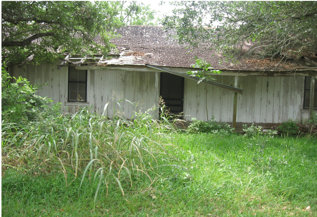
Figure 284. Street Number Unavailable, FM 445, Residence 2, looking east.
