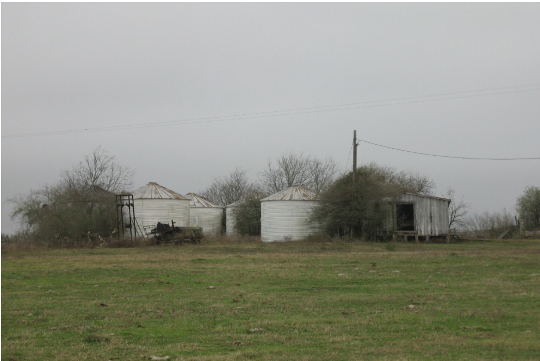
Figure 280. Street Number Unavailable, Cushman Road, Barn 7, looking south-southeast.
