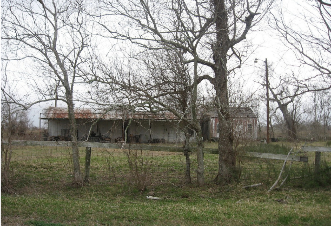
Figure 282. Street Number Unavailable, Cushman Road, Barn 8 and Residence 22, looking west-northwest.
