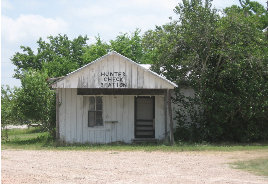
Figure 286. Street Number Unavailable, FM 445, Residence 4, looking southeast.
