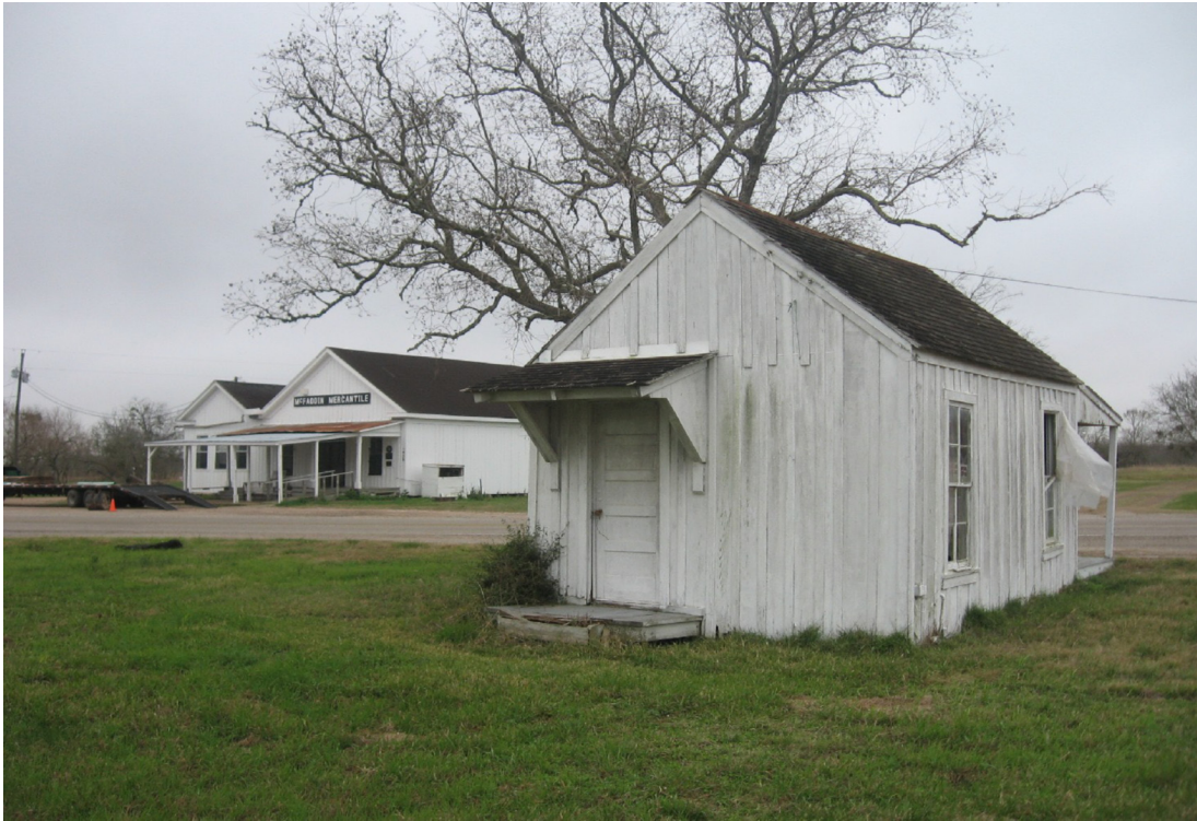
Figure 268. Street Number Unavailable, FM 445, Historic McFaddin Post Office looking southeast.
