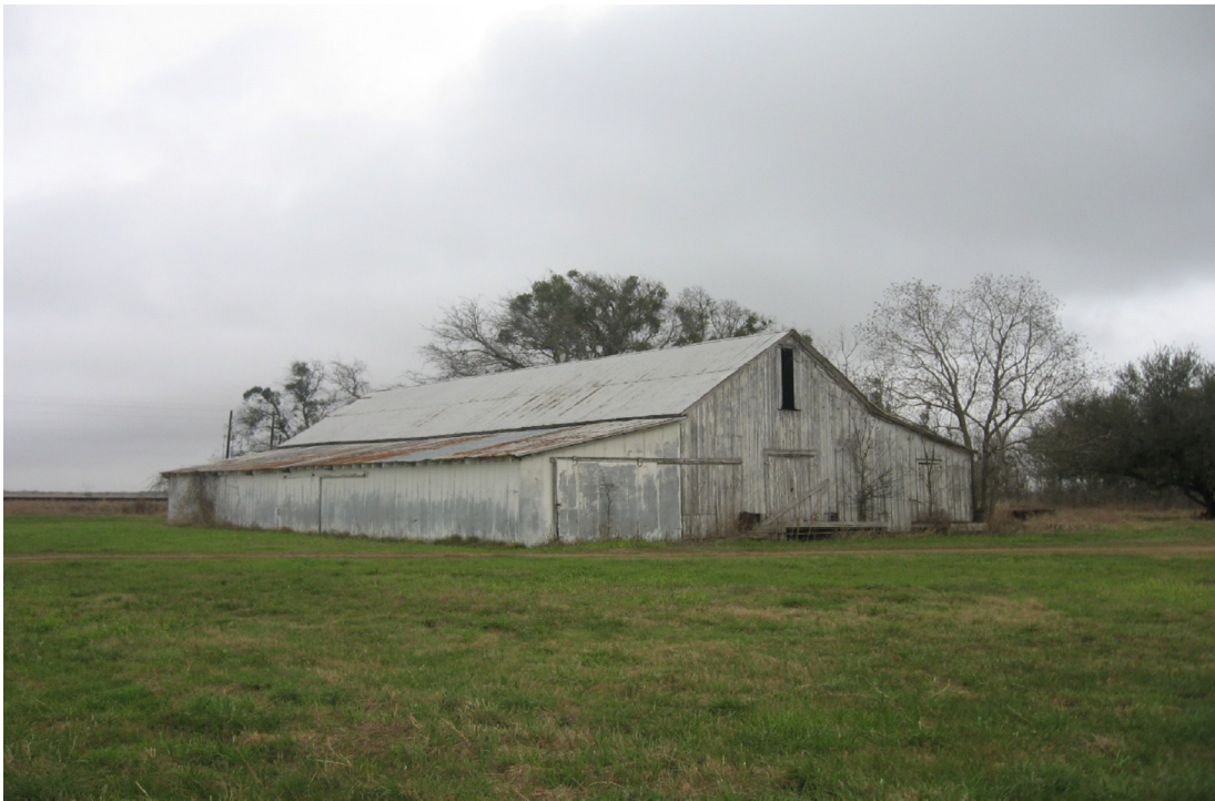
Figure 273. Street Number Unavailable, FM 445, Barn 1, looking northwest.
