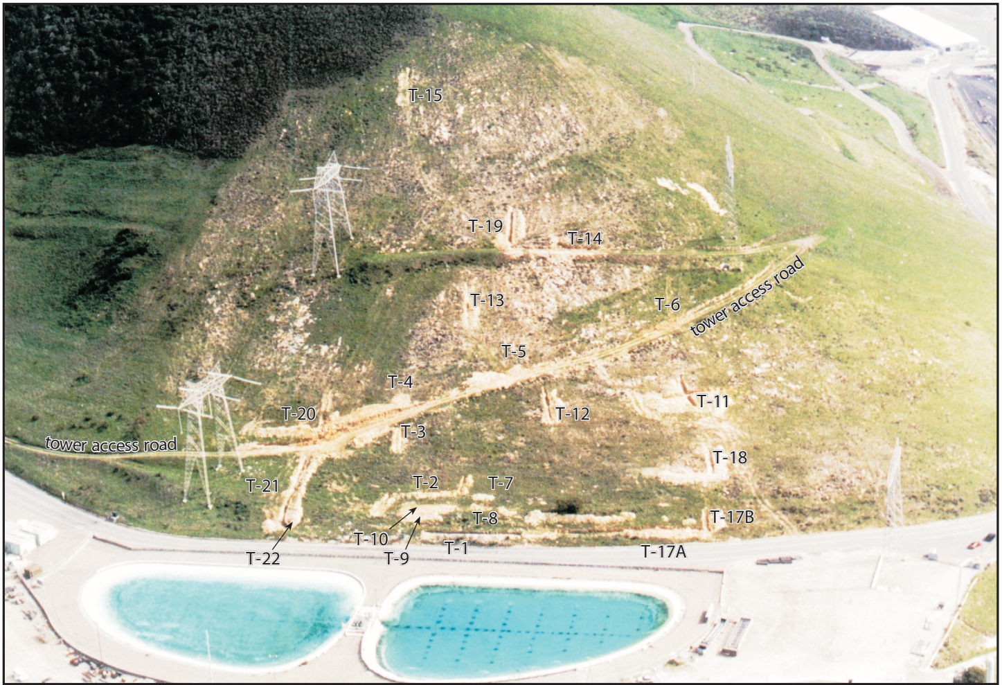
Southward view of the ISFSI site, above the raw water reservoir. The 1971 borrow area cutslope is indicated by areas of bedrock exposure and brown grass. Trenches excavated for the ISFSI investigations are shown (trenches backfilled in April 2001). Trench T-16 is located to the left of the photo. Photo roll AR 3-25.
