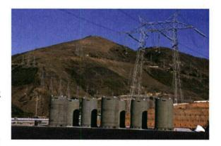
storage overpack that consists of 8 to 10 inches of steel or several feet of concrete (2 to 3 feet). The natural flow of air through the casks provides adequate cooling for the spent fuel inside.
