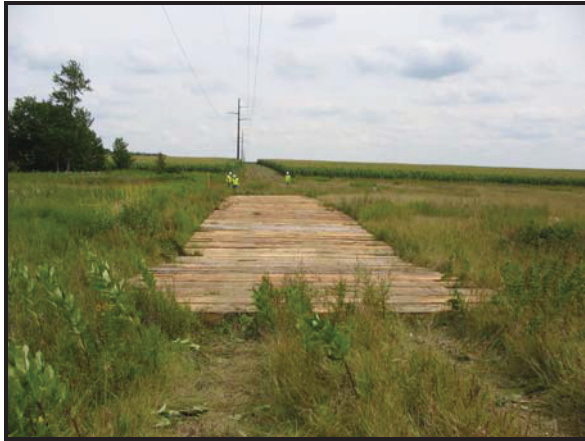
Figure 7 Mats Used in a Wet Meadow
