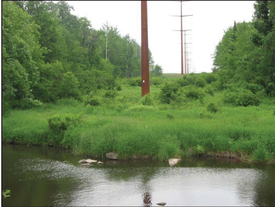
Figure 6 Restored River Bank Following Construction
