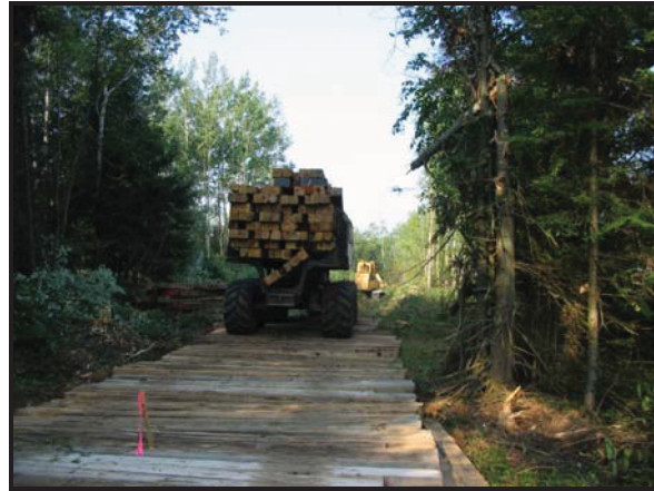
Figure 8 Mats Used in a Wooded Wetland
