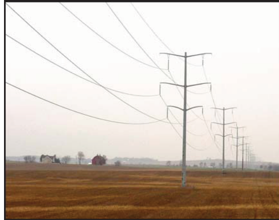
Figure 2 Typical Single-Pole, Double-Circuit Structure
