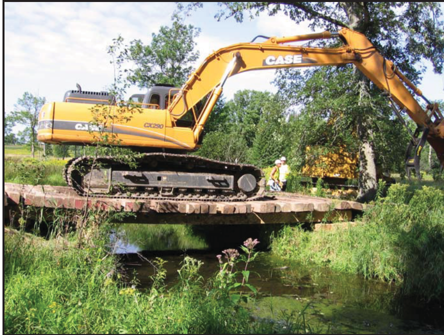
Figure 5 Temporary Bridge Structure Spanning a Waterway
