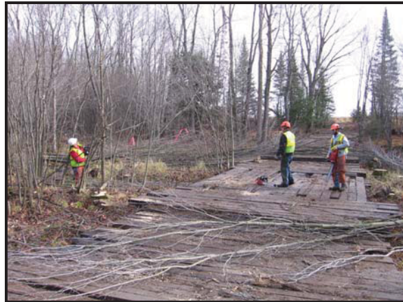
Figure 10 Hand Clearing Along a Flood Channel
