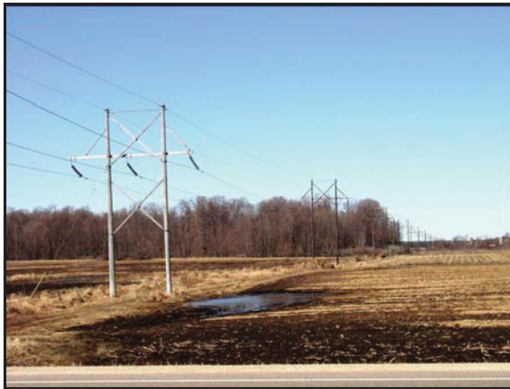
Figure 1 Typical Two-Pole, H-frame Structure
