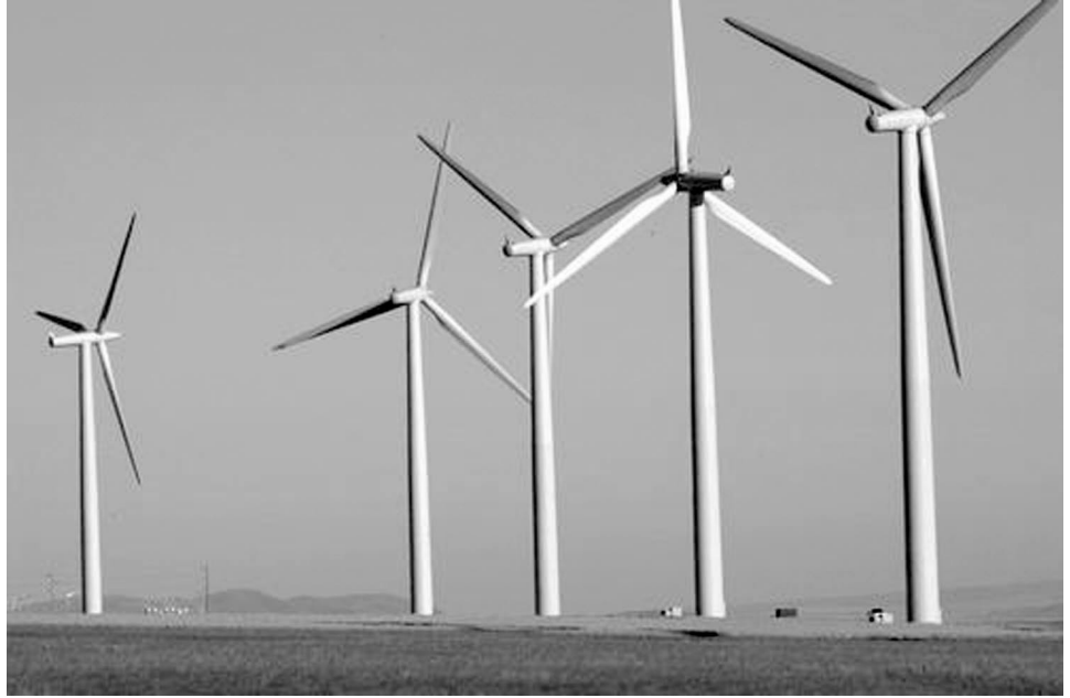
Figure 4: Example of a Newer Generation Wind Power Facility
