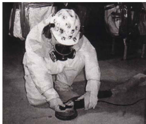
Concrete Grinder in Use Exhibit 3-8.
