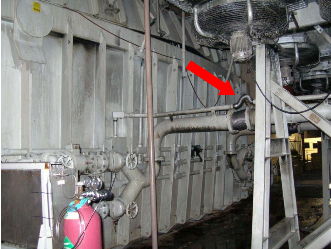
Fig. 6: Photo of external appearance of 21MT taken by IPEC personnel the night of the fault. Red arrow points to deformed conduit from force of explosion.
