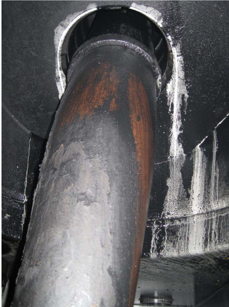
Fig. 13: Condition of the "A" phase HV bushing
