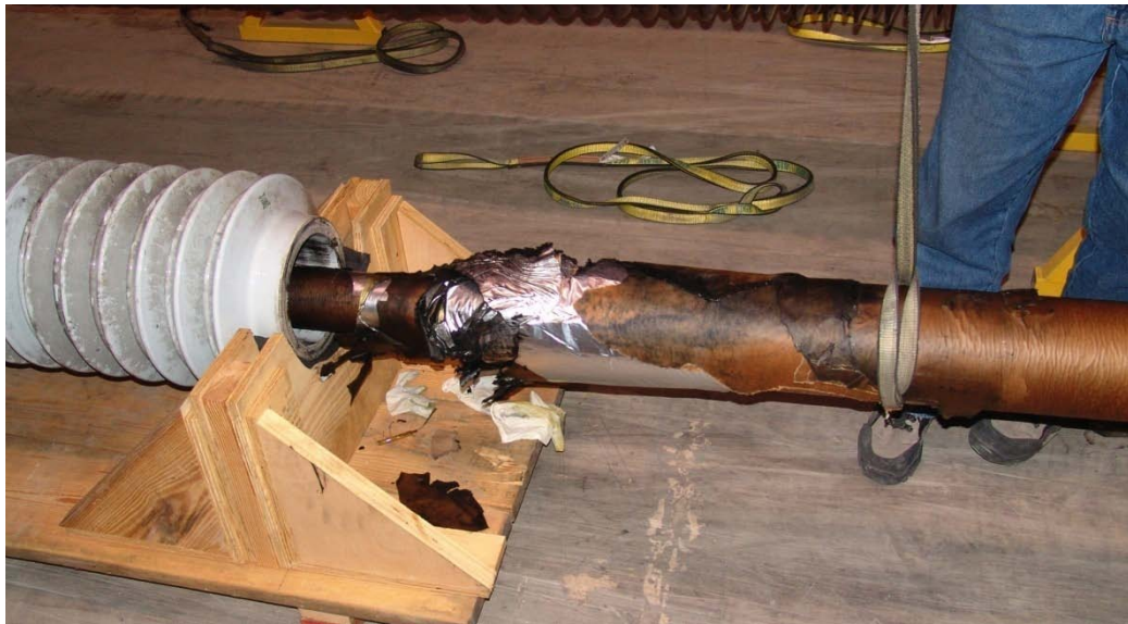
Fig. 16: Removal of core from bushing at Ajax Trench facility
