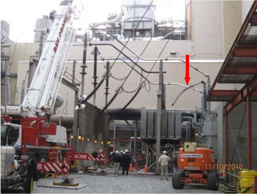
Fig. 7: Rigging crews on-site to disassemble 21MT. Red arrow points to fractured HV feeder bus section.
