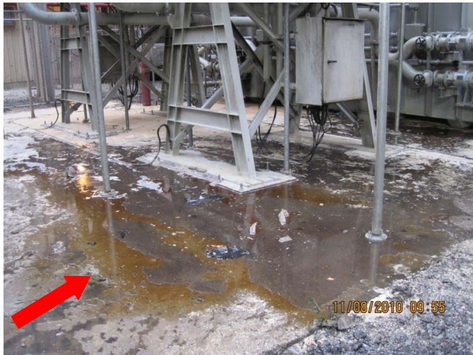
Fig. 5: Oil released following the 21MT tank rupture
