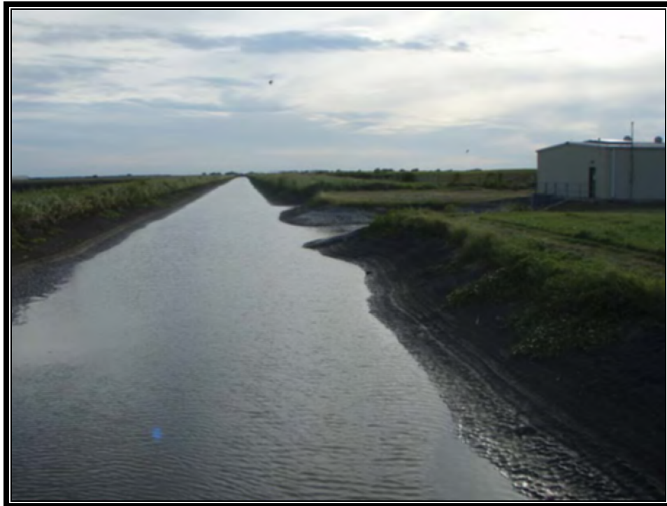
GBRA Main Canal with only a few inches of water in September
